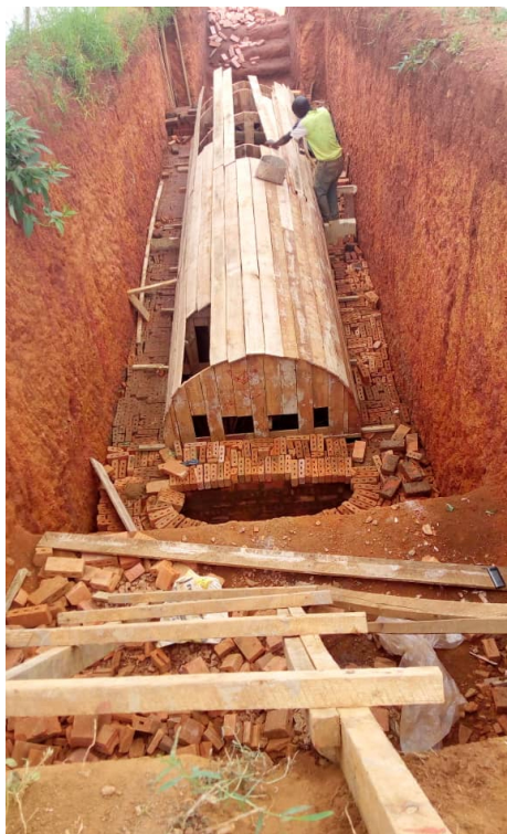
The underground in situ kiln under construction
