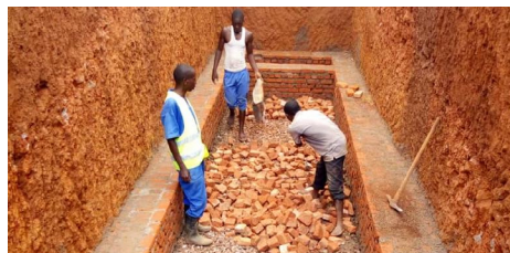
2. Underground kiln construction - 80 m 2
